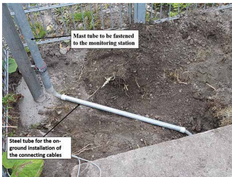
Figure 5. Installation of the connecting cables for the pull-cable switches.
