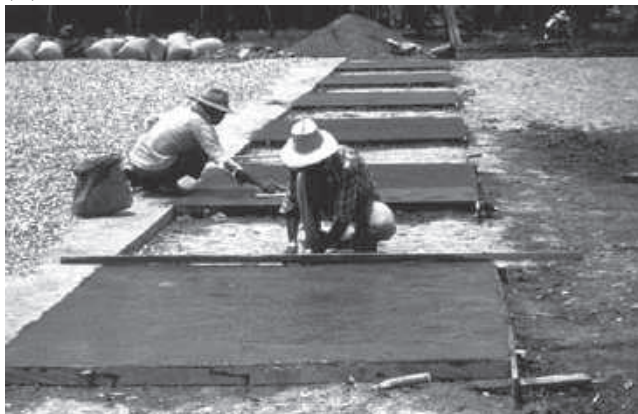
Figure 21-15. Expansion joints are placed between concrete slabs (A), together with iron rods (B).
